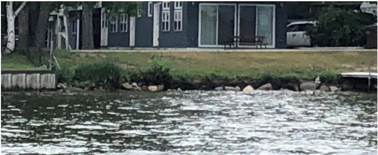
**Figure 28. Rip-rap failure due to wave action and high-water levels.**
